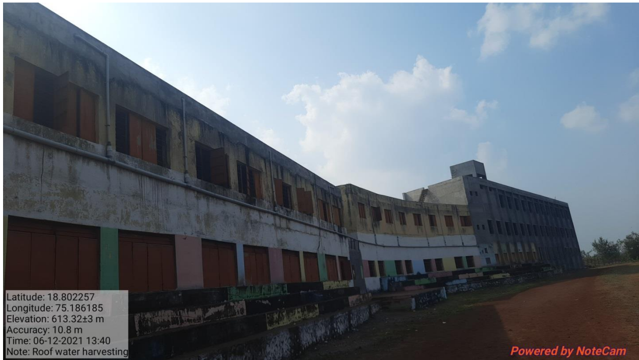
Roof water Harvesting
